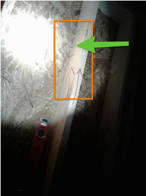
Exposed nails back left of crawl space stud. Right side of left rear pocket
