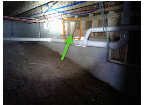
Exposed nails missing stud. Crawl space
