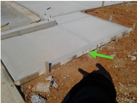
Front service walkway concrete forms still present . Unable to identify sides due to this
